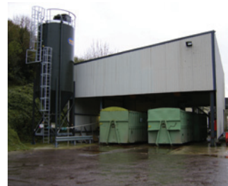
Lime silo and condition sludge container storage
