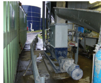
seepex BTI lime mixing pump
