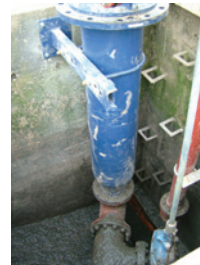
Desludge wet well
